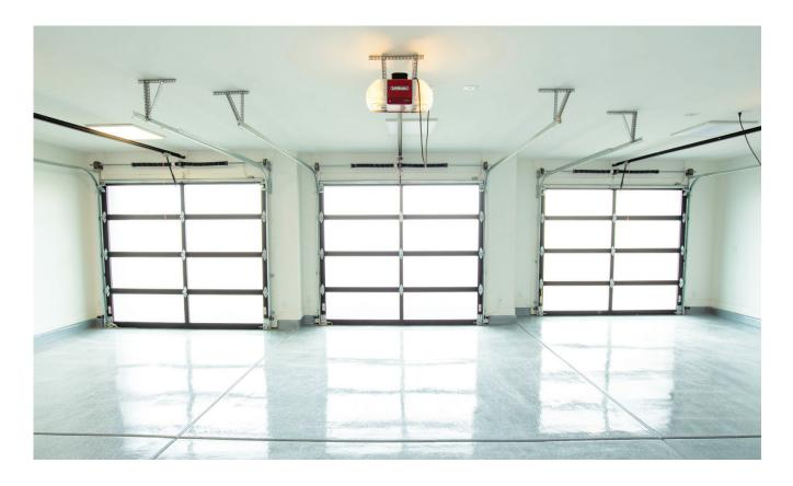
Inside the garages, Mandalay Homes has transitioned away from conventional 40-watt fluorescent tube overhead lights in favor of LED panel lights; the up-charge for those fixtures is mostly offset by their greater light output and improved light quality. An internet-controllable garage door opener from LiftMaster is also standard in the garage.
