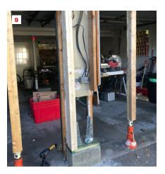
After letting the concrete cure, the author capped the footing with a treated 2x8 sill (7). He drilled and epoxied galvanized hold-downs into the concrete footing (8) and drove special lag screws to secure them to the bottoms of the new support studs (9).
