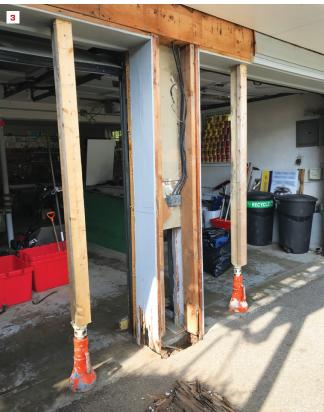
After being struck by a car, the garage support showed signs of internal rot as well as structural damage (1). The author peeled back the siding and sheathing to find that the support framing had been placed directly on top of an untreated 4x6 timber that had rotted (2). Before doing any more work on the support, the author propped up the continuous 6x12 header spanning the openings with a pair of house jacks (3).
