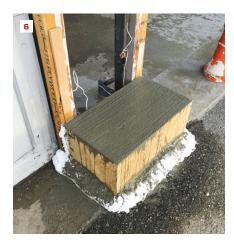
The author cleaned away the rotted wood, dug out the hole, and added a layer of crushed stone (4). He epoxied rebar into the garage slab as well as the aprons (5) before forming and pouring the concrete footing (6).
