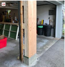
Solid 2-by blocks span between the studs on either side of the garage support to add rigidity (12). The treated sill had been kept back ½ inch from the face of the footing so the sheathing could be installed flush (13). The exterior of the support was finished with cedar shingles and PVC trim to match the house.
