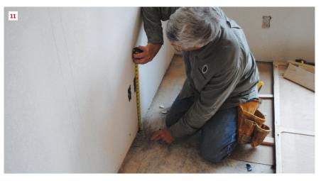
To reference electrical-box locations, the author plumbs down from each box with a level, marking the locations on the floor (10). Then he measures to the top and bottom of each box and marks the measurements next to the plumb marks (11). When the panel section is lifted into place, he merely reverses the process to locate and cut out the boxes.
