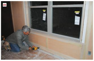
To let the horns of the window stool wrap onto the panel frames, the author installs the stool after completing the side panel installation (23). He then pads out below the window to allow the window panel to step out from the side panels (24). With the window panel nailed in place (25), the step-out detail adds a decorative accent when finished with baseboard.
