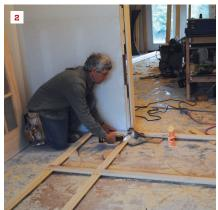
The author first draws a full-scale layout of the wall panels, getting proportions right and making sure electrical boxes fall in the field of the flat panels (1). Starting with the longest wall, he cuts and assembles the frames face down on the floor in front of where they'll be installed (2). Assembly moves along quickly with pocket-screwed joints, which don't require long clamps.
