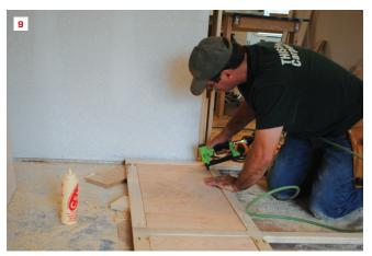
Instead of using a chisel to square up the rounded rabbet corners left by the router, the author just clips the panel corners with a miter saw (7). Before dropping the panels into the frame, a crew member carefully applies a bead of glue to the rabbet and spreads it thin to avoid squeeze out (8). Medium crown staples hold the plywood panel tight against the frame while the glue dries (9).
