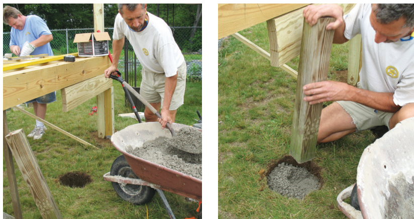
Figure 3. In a top-down framing approach, the deck is framed on temporary supports (above left), which allows for more accurate placement of the footings (above right). In some jurisdictions, the approach allows for a single inspection visit for framing and footings.
