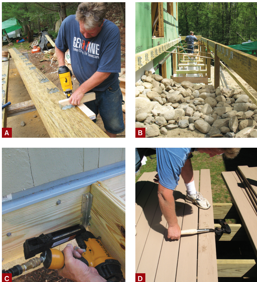
Figure 2. Joist hangers can be preinstalled on the framing, using a simple joist-hanging jig to accurately position the metal hardware (A). After the rim joist and ledger have been installed, joists can be quickly dropped into place (B). Key specialty tools include metal-connector nailers (C) and board benders (D).
