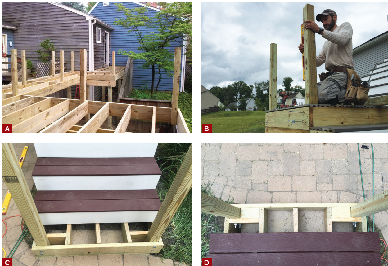
Figure 5. Tacking guard posts in place as the deck is framed (A), then going back later to install blocking and plumb the posts all at once (B) can help speed installation. Both vertical (C) and horizontal (D) blocking can be used to reinforce the connection between stair guard posts and the stair stringers, though remember that blocking installed on the flat should be protected from water intrusion with a peel-and-stick flashing membrane.
