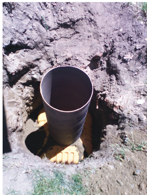
Figure 1. Some building inspectors may allow you to skip certain jobsite inspections as long as you can provide them with clear photos showing that your work meets local code requirements, such as footing depth (top). Not having to wait for the inspector will keep the job moving. Another benefit to taking photos is that you will have documentation of the details used in the construction of the deck (right).
