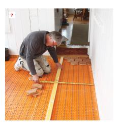
A crew member does a dry layout across the floor, adjusting the grout joints for an even layout (5). To set the starting point for the installation, he scribes the tiles that will be installed at the main doorway into the house (6). Before installing the tile, he measures from the wall to keep his installation guide—a long level—parallel with the wall (7).
