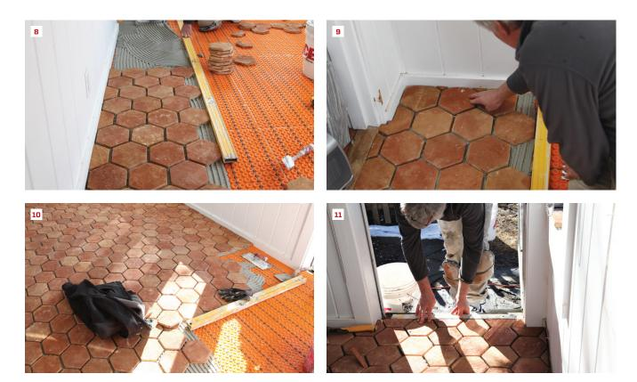
After spreading unmodified thinset with a 3/8-inch notched trowel, a crew member installs the tile using the level as a straightedge against the outermost course (8). In the corner, he scribes and cuts the jamb profile at a closet doorway (9). All cuts are made with a wet saw. Switching to a shorter straightedge, he works his way back across the room (10). A short strip of wood aligns the last tiles at the entry door (11). A threshold will be installed later to protect the tile at the entry.
