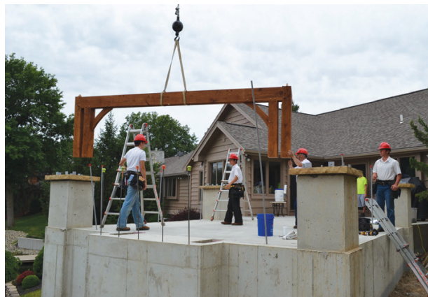
Once the components have been assembled on the ground, a crane lifts them into place, where they are installed by the OakBridge team.
