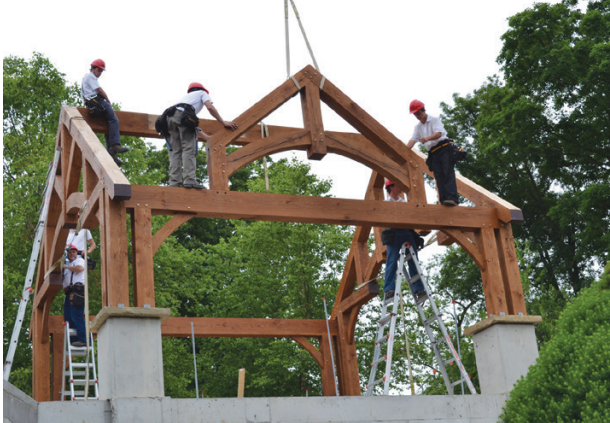
After OakBridge workers installed the dormer face truss and remaining 8x8 rafters to finish up the frame, a local crew installed a white-pine tongue-and-groove roof deck.
