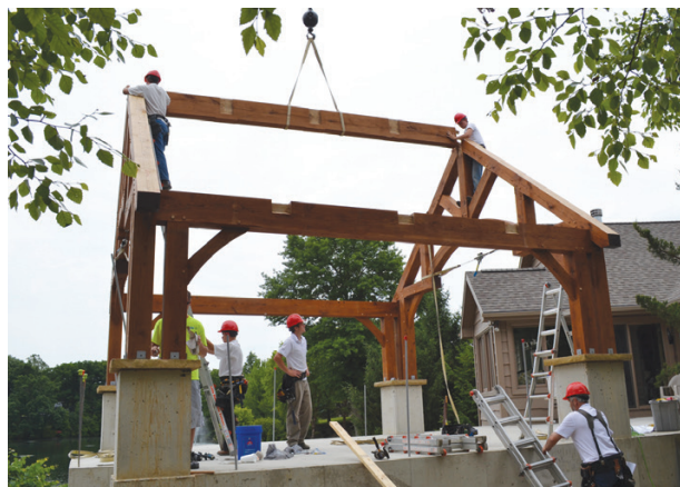
A 6x12 ridge beam ties the two end trusses together. For temporary protection, the pieces were coated with a water-based finish back at the woodshop.
