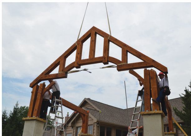
Crafted from 8x8 white-oak timbers with 8x12 plates, the 18-foot-wide frame has a 10-in-12 pitch roof. Above, a king post-and-strut truss is being lifted into position.
