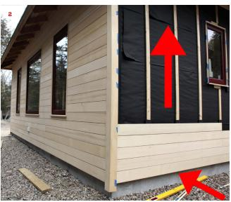
**Drain and dry.** A rainscreen is an air space between the cladding (siding) and the water-resistive barrier (WRB). In these examples, the rainscreen is created by attaching the cladding to furring strips fastened to the wall framing. The red arrows in the left-hand photo (1) show the direction water drains—down and out—through the space via gravity. Just as important, a rainscreen allows air to enter to dry out both the WRB surface and the reverse side of the cladding (2).
