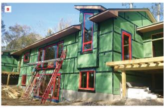
Closed vs. open rainscreen. Wood clapboards are an example of a closed rainscreen system, where each layer of cladding laps over the layer below (7). All the ventilation in a closed system comes via the openings at the bottom of the rainscreen. In an open system, gaps between the siding boards allow increased ventilation to enhance drying (8). Before rainscreen is installed, the building should be 100% airtight, weathertight, and water managed (9).
