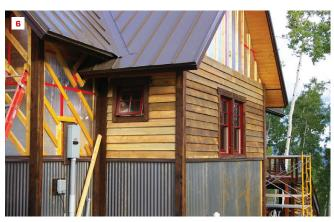
**Manufactured or site-built.** The most common type of manufactured rainscreen is a mesh that attaches between the cladding and the WRB (3). Vertical furring strips are a good way to create a rainscreen space (4). Screening at the bottom of the space keeps out pests (5). For vertical siding, furring strips can be mounted on the diagonal to allow for drainage (6).
