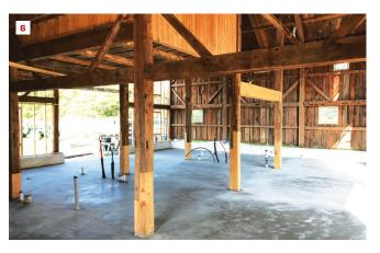
The barn's original frame and board siding had more charm than integrity (1). To expose the foundation, the barn was jacked up and moved back off its location (2, 3). Thick concrete pads were placed to support the interior post ends (4), and a concrete perimeter foundation was placed (5) to elevate and support the walls. Inside the building, posts needed to be spliced for length, as well as to replace the deteriorated post ends with sound material (6).
