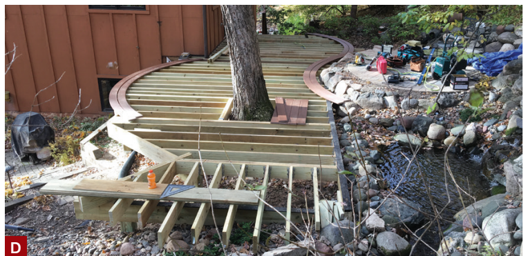
Figure 1. The author installed cantilevered joists over dropped beams, running the joists long (A) and then laying his heat-formed borders over the joists (B) to define the curves. After the joists were marked and cut to length, workers installed blocking as needed (C) and framed the opening around the tree trunk (D).
