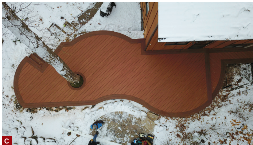
Figure 3. The author screwed black plastic pipe to MDF backing to make the form for the 16-inch-diameter trim ring around the tree well (A, B). It took two workers to pry the ends of the trim ring apart as they slipped it over the tree trunk, like putting a key on a key ring (C).
