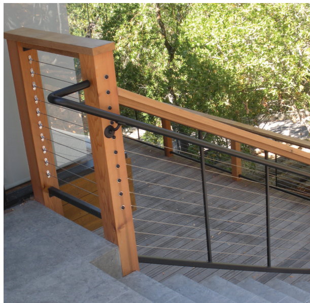
Figure 7. Surface-mount fittings are useful when access to the back of a post is limited or where the cable terminates at a wall.
