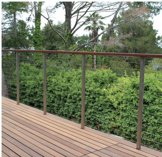
Figure 6. The author often combines wood top rails with aluminum- or steel-framed rail systems. To maintain the cable spacing, posts and intermediate pickets should be no more than 3 feet apart.
