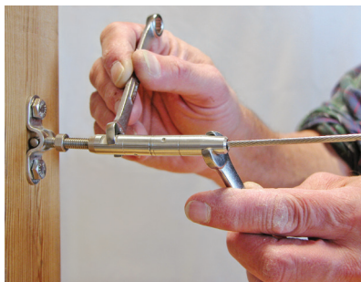
Figure 1. Typical of other swageless fittings, Feeney's Quick-Connect fittings have locking jaws that grab the cable without requiring the use of a swaging tool. After the cut end of the cable has been inserted into the fitting, a pair of wrenches are used to tighten the fitting and tension the cable (above left). A crimping tool (above right) is needed to attach swaged fittings to cable.
