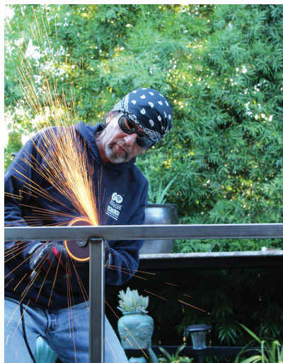
Figure 4. The author fabricates his own stainless steel frames; here, he's smoothing a welded joint (above left). His shop is equipped with simple jigs that allow him to accurately weld mounting plates and drill holes through the tubing for the cable (above right).
