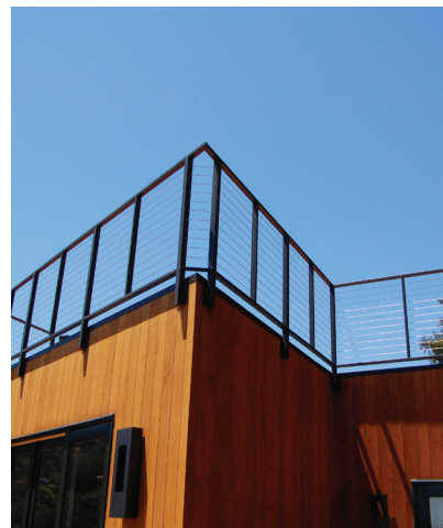
Figure 3. To gain a little extra square footage, fascia-mounted wood posts (above) or steel posts (above right) can be lag-screwed or through-bolted to the framing. Fascia-mount brackets for wood posts are also available.
