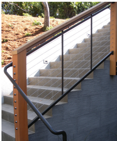
Figure 3. To gain a little extra square footage, fascia-mounted wood posts (above) or steel posts (above right) can be lag-screwed or through-bolted to the framing. Fascia-mount brackets for wood posts are also available.
