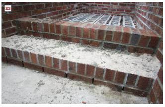
**Weep holes for drainage.** To provide drainage, the author left the head joints in the lowest course of the stairs unmortared, with sand keeping the bricks behind that course clear of mortar droppings (22). A rowlock course finished that step, leaving the open weep holes, and he spread a layer of sand to protect the step from mortar droppings as he worked his way to the top (23).
