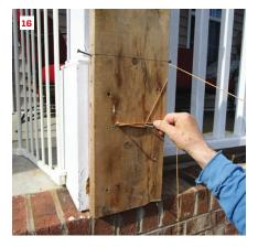
**Stringing the slope.** With the first angled brick placed, the author set up two lines to follow as he laid up the sloping side walls of the staircase (14). At the bottom, he held the lines with a 2-by block ripped to 29 degrees (the layout pitch) (15). At the top, he attached the lines to the sides of a board ripped to  $7^{5}/8$  inches (the width of the wall), anchoring them to a makeshift cleat (16).
