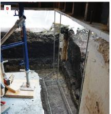
The new footing was reinforced with 1/2-inch rebar, which was tied to chairs pinned to the base of the footing trenches (8). The rebar in the footing was wired together with vertical rebar that extended up through holes in the existing sill plates (which would later be replaced), tying the footing to the concrete-block replacement foundation (9).
