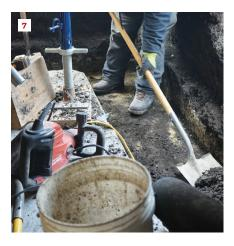
The foundation walls in this corner were in bad shape and fell apart easily with an impact hammer (5). Once the walls were removed back to solid concrete, excavation for the footings could begin (6). The crew dug trenches 12 inches deep and 24 inches wide for the footings, removing all the excess soil and debris in five-gallon buckets (7).
