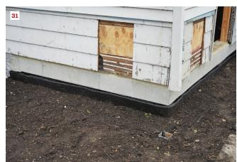
To finish the exterior of the new foundation, the crew applied waterproofing to the block, after first masking off the part of the block wall that would extend above grade (27). Removing the tape left a clean line on the block (28). Then they secured drainage mat to the block with concrete fasteners (29) and backfilled with pea gravel to provide additional drainage next to the mat (30). Once the topsoil was in place, the only remaining task was repairing the beam holes in the siding (31).
