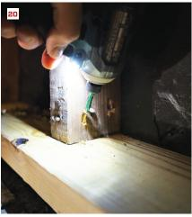
With the block wall finished, the crew replaced the old sills with new treated sill stock (19). Using inflatable shims and heavyduty pry bars to hold the new plates tight against the bottoms of the existing studs for fastening, the crew then drove galvanized toe screws through each stud and into the sills to secure the sills to the studs (20).
