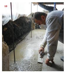
With limited space and limited exterior access, the crew had to mix all the concrete by hand (10). Each batch was dumped into the trench until the footing was level with the basement floor (11). To remove air bubbles and create the densest concrete for the footing, the crew vibrated the wet concrete (12). Vibration not only consolidated the concrete but also made the mix more liquid, which made it easier for the crew to smooth the wet concrete surface of the footing with a float (13).
