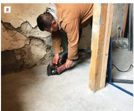
To help support the house walls at the corner, the crew bolted LVLs to the studs (1). A crew member scored the concrete with a saw for the new footing (2). After making holes in the sheathing, the crew inserted needle beams and supported them inside with double screw jacks (3) and on the exterior with solid cribbing (4). The beams supported the exterior walls via the LVLs.
