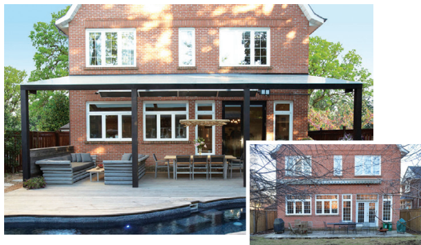
The original exterior (inset) was updated with a new terrace door and the addition of a sandblasted tempered-glass roof to shelter the outdoor dining and living areas.
