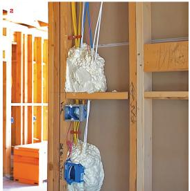
In a typical one-story garage attached to a two-story home, the roof ties into the second-floor walls; in this case, into the knee walls of a much larger attic area. Below the rim joist, the author's crew hangs drywall on the garage side of the wall, ahead of the drywall crew that will install drywall in the rest of the house (1). This allows him to begin air-sealing penetrations, such as packing electrical boxes with a two-part, closed-cell spray foam (2).
