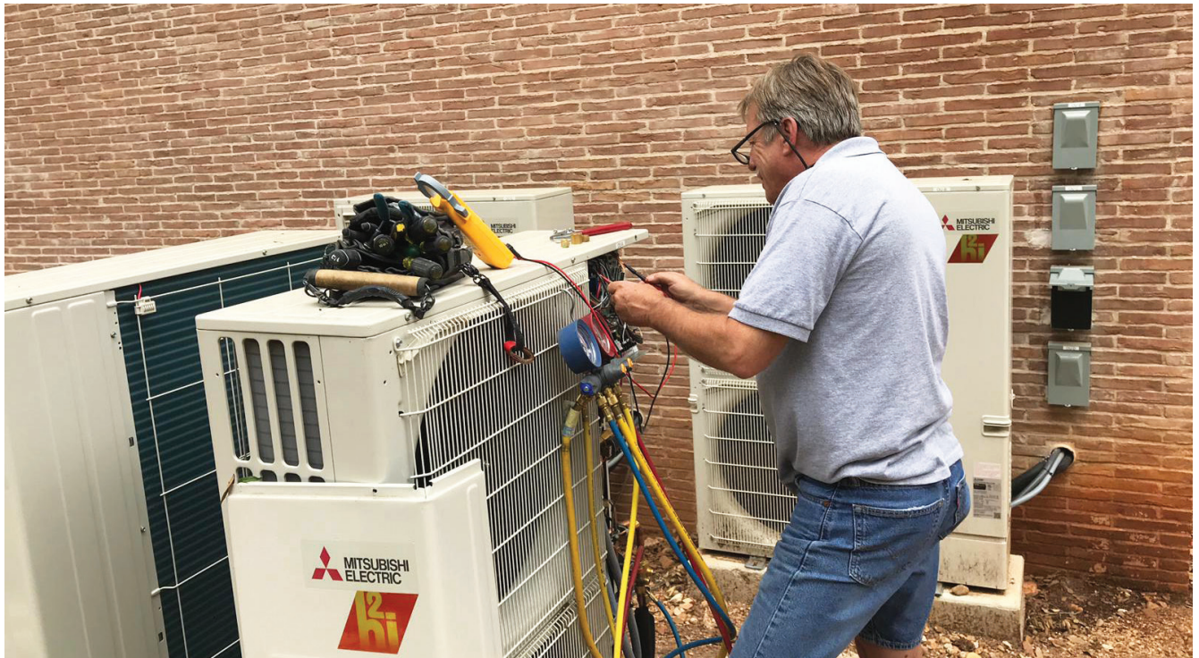
Gilbert Rosipal of Air Rite By Design of Austin, Texas, wires up a Mitsubishi variable refrigerant flow (VRF) outdoor unit. Controls in the compressor allow the system to ramp its power up and down gradually, dialing back to as low as 15% of full capacity when appropriate to address “part-load” conditions.
