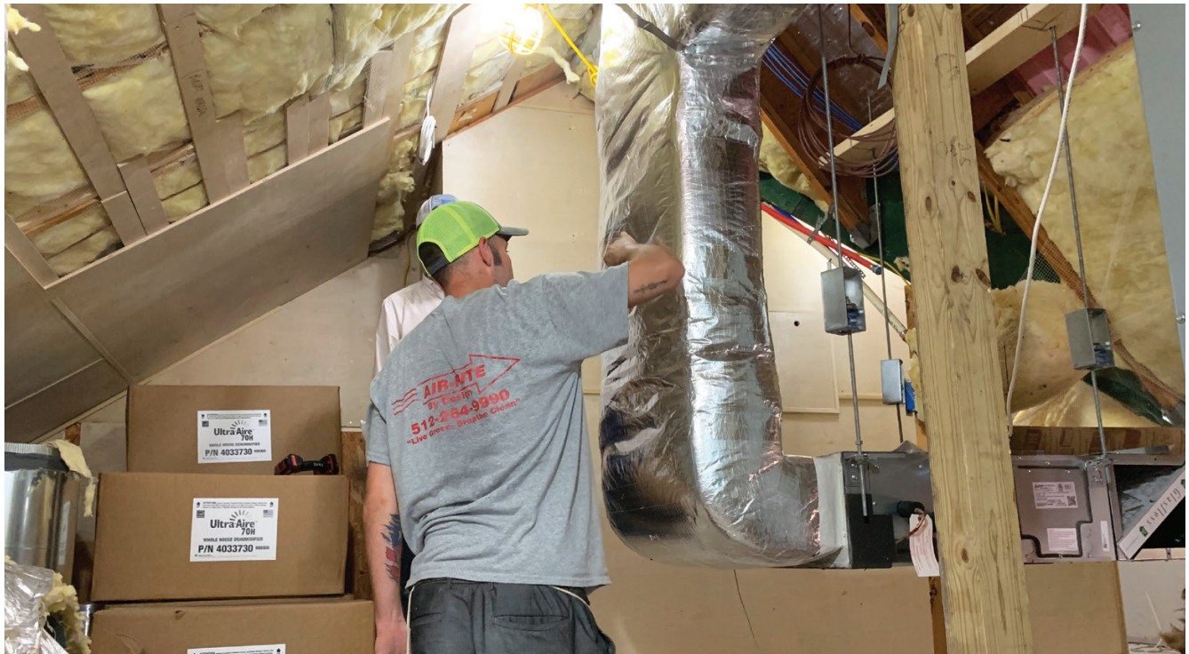
An installer for Air Rite By Design tapes insulation on a duct. Even though the ducts are within the conditioned envelope, they still must be insulated. At right is a multi-position air handler for a variable refrigerant flow (VRF) system. The air handler is suspended from the roof framing with threaded rod and vibration-damping couplings.
