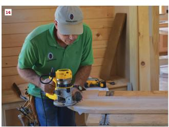
The author measured and cut the upper blank to fit around the skirt boards before scribing the radius (11). After projecting the edge of the radius out  $2^{1}/4$  inches as with the lower step, he cut the curve with a jigsaw (12). For both steps, he used a belt sander to smooth out the curves (13) and then routed a bullnose into the edges using a round-over bit (14).
