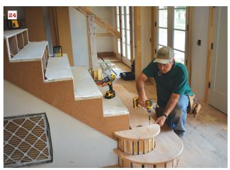
After applying a liberal amount of construction adhesive to the rough tread (21), the author set the finished upper tread into place (22). As before he plotted out the exact fastener location with a framing square (23). He then drilled and drove finish-head screws at each location (24). Each starter step was held in place with four pairs of screws.
