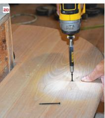
Sanding the rough treads prepared them for the finish step installation (15). After applying adhesive to the rough step (16), the author set the finished lower step in place (17). He plotted out the exact fastener locations with a framing square (18) and then drilled straight-sided holes (19) for the finish-head screws (20). The floor finishers later filled the holes and stained the steps.
