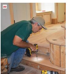
For the step down to the lower level, the author templated the curve out of 1/4-inch plywood (25). After positioning the template on the blank and plotting the curve (26), he cut the curve with a jigsaw (27). He routed a bullnose where the step returned to the riser (28), and he bedded the finished tread in adhesive (29). Finish-head screws completed the installation (30).
