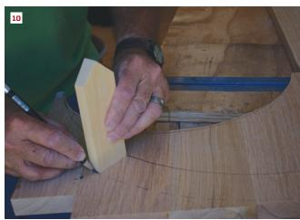
The author set the lower blank atop the upper riser to scribe the inside radius (7). After cutting the inside radius with a jigsaw (8), he set the blank in position on top of the lower riser and scribed that radius (9). To project the scribe line to the desired overhang, he followed the line with a  $2\frac{1}{4}$ -inch block of wood (10) and then cut the outside radius to that line.
