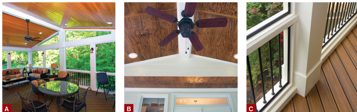
Figure 4. When planning ceiling finishes, keep in mind how light fixtures and ceiling fans may affect the design (A). It may be necessary to incorporate structural features of the existing house, such as this second-floor cantilever, into the porch ceiling (B). Shown here is the author's standard sill plate, chair rail, and column detail, all executed with PVC trim (C).
