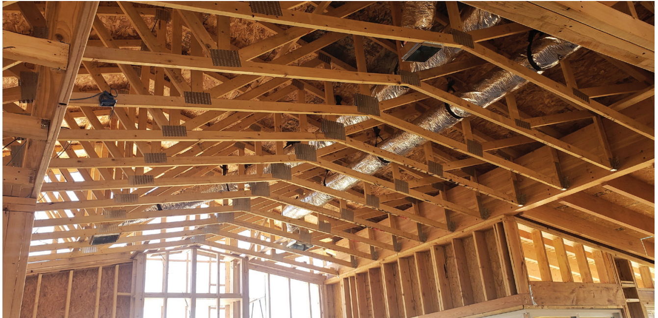
The home's HVAC duct system delivers conditioned fresh air to every room in the house. A centrally located return pulls stale air from the living space and exhausts it to the outdoors.
