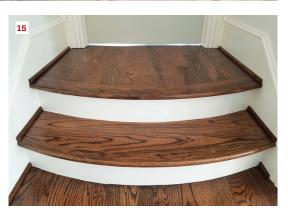
To rough-fit the tread, the author scribed an arc 11½ inches from the outside arc (11), fine-tuning the fit after setting the tread in place (12). After scribing and cutting the ends of the tread for the skirtboard (13), he applied glue to the rough step and screwed the tread into place (14). Then he made the curved nosing for the top step, which was installed by the flooring contractor (15).
