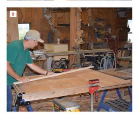
Using the formula shown in the illustration (right), the author calculated the radius of the lower step roughed out by the framer (1). With the stair blank clamped to the bench, he found the center point using a trammel beam set at the radius (2). He then scribed the arc on the blank to be sure that it fit properly (3).
