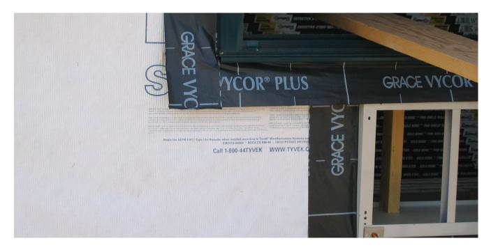
Flashing should be applied so as to direct water out and down on the drainage plane. Weep screeds at the bottom of the wall allow any water that soaks into the plaster to escape.
