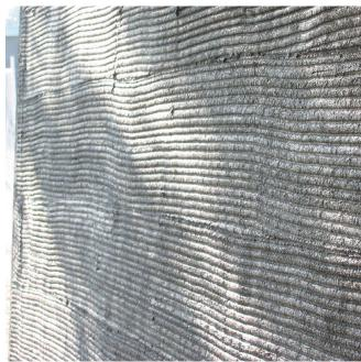
Above left, an inferior scratch coat does not fully cover the wire lath and has not been properly cured, allowing the coat to scale away from the wall. Above right is a superior scratch coat that fully covers the lath and has been scored (scarified) to create grooves that will provide a mechanical bond with the brown coat.
