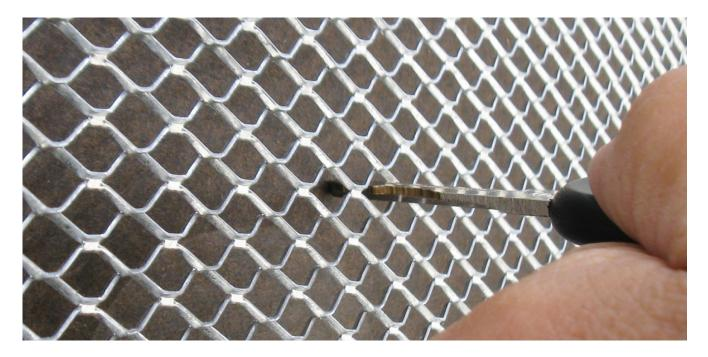
Wire or mesh lath should stand proud of the drainage plane by 1/4 inch. This allows space for the scratch coat of plaster to fully embed the lath. The scratch coat should cover the lath by another 1/8 inch.
