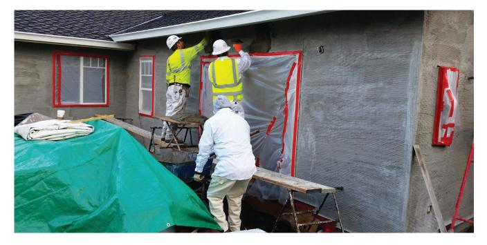
After the scratch coat has been moist-cured for at least 48 hours, the brown coat is applied with firm pressure to create a strong mechanical and chemical bond between the coats. The brown coat should be rodded flat with a darby and straightedge, then moist-cured and checked for hardness.
