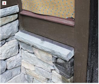
With a porous stone like bluestone, the process of spalling (also called "thermalling" or "flaming") can be used to rough up smooth-cut surfaces. After thoroughly wetting the stone (1), the mason applies heat with an acetylene torch (2). The heat turns the water to steam. The rapid expansion of the water causes the outer layer of stone to pop off (3). He repeats the wetting and heating process until the desired amount of spalling is achieved.
