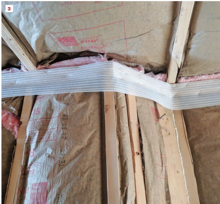
Here, the builder has applied sill-sealer material to the top plates in a home (3, 4). When drywall is installed, the sill sealer will form a gasketed seal and prevent air infiltration at the top of the wall.
