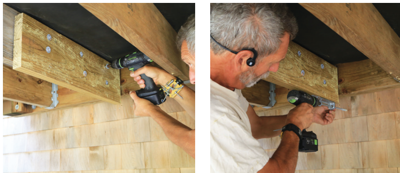
Figure 10. Blocking can be installed to help align the hardware with the deck and house framing. Here, the author fastened the block to the joist with SST TimberHex HDG screws (above left) before installing the DTT1 tie (above right).
