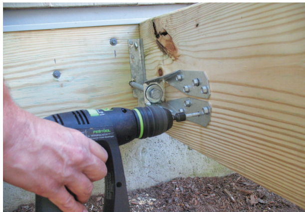
Figure 3. When deck and house joists are parallel, screw a metal tie to the side of a house joist and another to a deck joist with structural screws, drill a hole for a 1/2-inch-diameter connecting rod, and bolt the two ties together.
