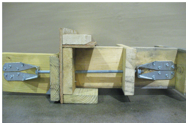
Figure 5. When house joists are perpendicular rather than parallel to the deck joists, solid blocking must first be installed between at least two joist bays, starting at the rim joist, then the tie must be mounted on the block furthest from the rim joist.
