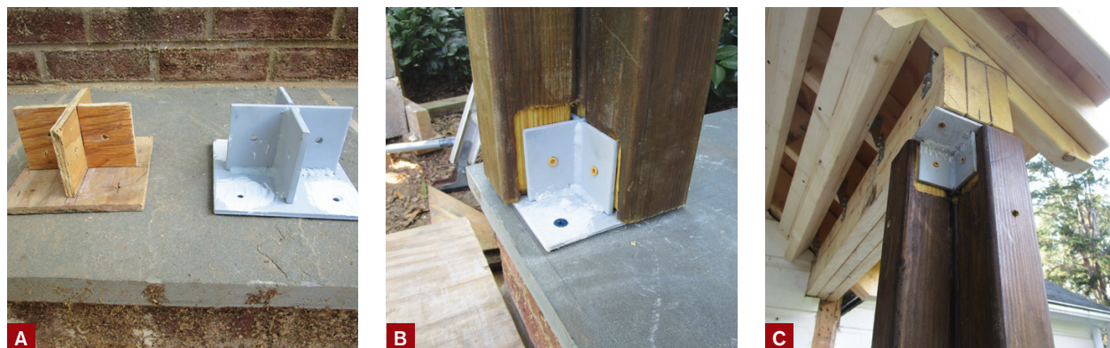
Figure 5. A local supplier fabricated the custom steel column brackets based on a plywood prototype supplied by the author (A). Each column consists of four 3x3 posts connected via the brackets to the masonry stoop (B) and beams (C).
