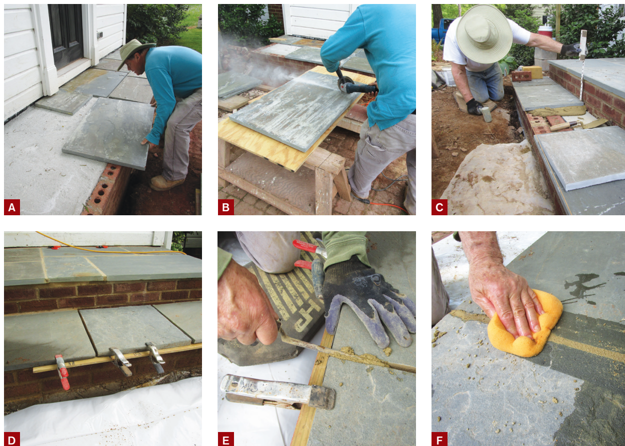
Figure 2. The author dry-fit the bluestone pavers (A), numbering them to keep track of their location, then trimmed them to size as needed with a diamond blade mounted in an angle grinder (B). The pavers were set in a thick bed of type S mortar (C). After the mortar bed cured, he grouted the 1/2-inch-wide joints with the same type S mortar. A strip of wood clamped to the pavers where they overhung the brickwork supported the grout while it cured (D). The author used a tuck pointer to pack the joints (E), and he cleaned up the joints afterward with a damp sponge (F).
