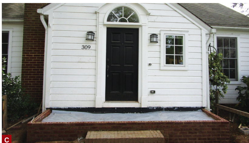
Figure 1. To expand the original front entry (A), the author removed its concrete slab deck and laid up a pair of block walls faced with brick on either side of the masonry stoop (B). Before pouring a new slab flush with the brickwork, he installed vinyl flashing to serve as a vapor barrier between the concrete and the mudsill and primed the cut edges of the siding and trim (C).
