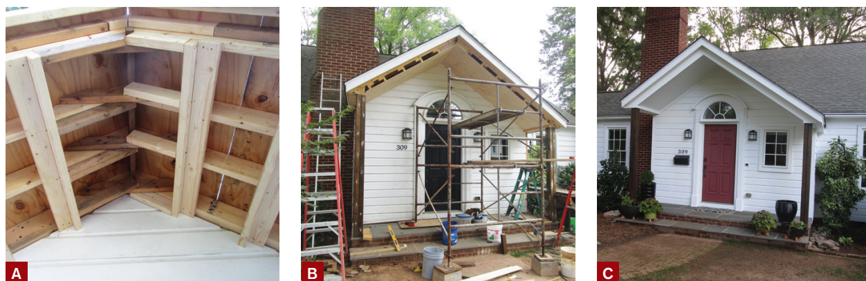
Figure 6. The author fastened collar ties to the rafters and ridge with structural screws (A) and blocked out the roof framing with 2x4s to provide nailing for the plywood ceiling (B). The completed portico was painted to match the house (C).
