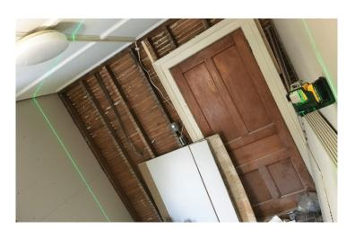
The author illuminates premarked stud locations by rotating the laser to each stud. No more marking the wallboard with level and pencil to minimize misses.
