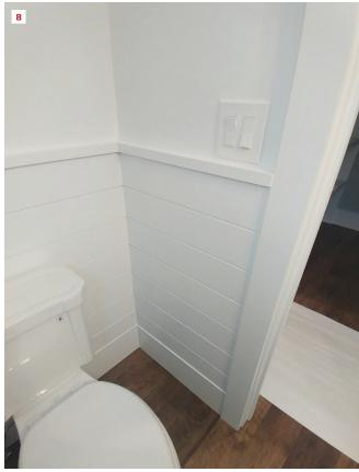
The author plans layout to avoid "slivers," or narrow lengths, at the top or bottom of a horizontal run when installing shiplap within a shelving unit (7) or as wainscot (8).
