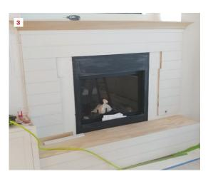
Figuring out how to terminate runs and make transitions is one of the first things to get a handle on when adding shiplap siding to a room. At outside corners, the author typically butts the shiplap into either square or rabbeted stops (1). To terminate a run of shiplap in the field, the author uses mitered returns cut flat on a sliding compound miter saw to hide end grain (2, 3).
