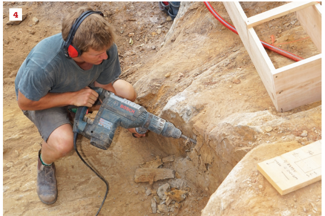
Crew members Finn Bradenday and Jackman Wood screw batter boards to trees at the low end of the sloped site (1). Lead carpenter Mark Pollard takes a measurement along a string line (2). Bradenday removes rock using a wet saw (3) and a rotary hammer (4) at a pier location.
