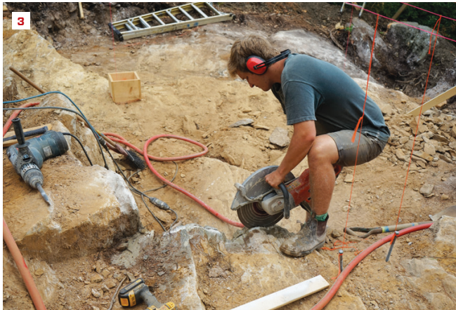
Crew members Finn Bradenday and Jackman Wood screw batter boards to trees at the low end of the sloped site (1). Lead carpenter Mark Pollard takes a measurement along a string line (2). Bradenday removes rock using a wet saw (3) and a rotary hammer (4) at a pier location.
