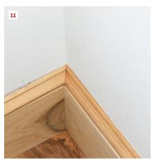
For base cap molding, begin by cutting across the profile from the bottom **(6)**. After cutting in from the end **(7)**, cut the curve working side to side **(8)**, then cut the top profile **(9)**. Sanding fine-tunes the cope **(10)** for the final tight fit **(11)**.
