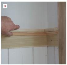
Before coping a joint, cut the molding at 45 degrees to reveal its profile (1). For cove molding, first cut in from what will be the vertical face (2), then cut in from the horizontal side (3). Because the miter will not be readily visible, the carpenter opts for a square cut on the horizontal side. He then follows the profile until the cuts meet, keeping the saw at an angle to create a back bevel (4). Giving the end of the coped trim a slight tap helps to close the joint for the final fit (5).
