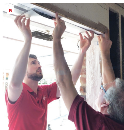
Some openings were prepped by filling the gap between the brick and the wall framing with gun foam (3), and caulking over the rough jambs (4). Site-bent coil stock was used at the head and sill of the openings (5) to direct water out to the face of the exterior.
