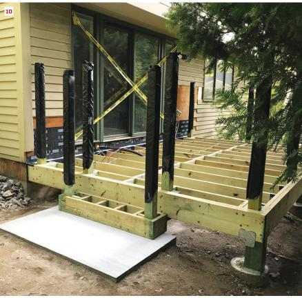
To help true up guard posts and lock them into position during installation, the author uses composite shims (9). Then he wraps the posts with garbage bags, which help prevent the posts from warping and twisting by protecting them from exposure to moisture and UV rays (10). Taping the bags tightly around the posts helps them to last until it's time to finish the railing system.
