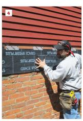
When modifying PT deck framing, follow cutting, notching, and drilling guidelines to avoid weakening the framing (1), and always treat end cuts and notches with an approved preservative (2) to avoid compromising the wood's rot resistance. The author uses 6x6 posts, which can be notched, to support all of his deck framing (3). Before installing a deck ledger, the author removes the siding and protects the sheathing with a layer of peel-and-stick flashing membrane (4).
