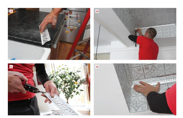
The author used tin crown embossed with an egg-and-dart pattern as an accent between the tray field and the perimeter (9). Because the molding was flexible, he used a combination square to set the height (10). Corners were coped much like wood molding, with snips cutting the curve of the cope (11), to create seamless inside corners (12).
