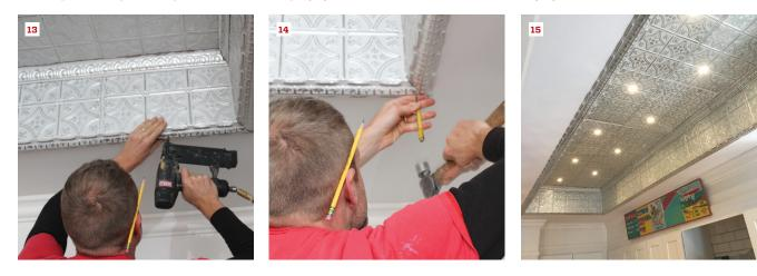
To finish the bottom edge of the tray ceiling where it returned onto the main ceiling, the author installed embossed picture-frame molding, making sure that the fasteners hit solid nailing (13). He used a nail set to drive all the fasteners to a proper depth without denting the tin (14). After finishing the tin installation, lighting was installed to complete the tray ceiling (15).
