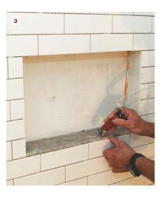
To waterproof a tiled niche, apply waterproof backerboard to the inside surfaces of the niche (1). (The back wall of this niche was in two pieces to facilitate installation.) Next, apply waterproof membrane, bedding it in unmodified thinset (2). With the waterproofing complete, install the tile starting with the bottom of the niche, which should have a slight pitch for drainage (3).
