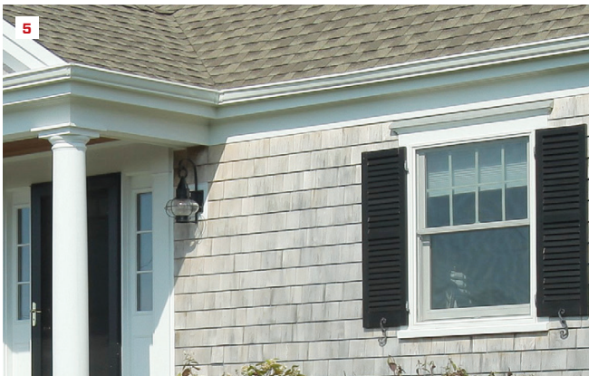
A frieze board (5) captures the top edge of the siding while closing the joint between the soffit and the wall.
