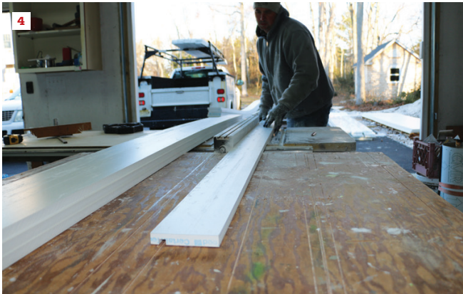
To join the fascia to the soffit, this crew member runs the 1-by fascia material through a table saw to create a dado groove (4).
