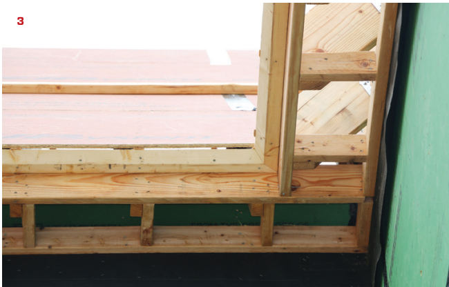
Seen from below, blocking between the subfascia and the wall adds plenty of nailing surface for attaching a wider soffit (3).
