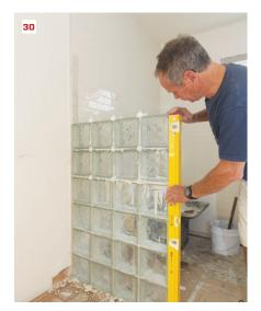
The author continues to check the glass-block wall every two or three courses for level (28) and plumb (29), as well as checking the end of the wall for straightness and plumb (30). He also adds panel anchors every two courses for the entire wall.
