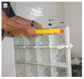
After installing the third and fourth courses (20), the author rechecks the glass block for level (21). He also checks the wall for plumb, making sure the block is also level across its width (22), as well as in plane (23). At this point, he scrapes the excess mortar out of the joints and lets the wall sit overnight to allow the mortar to cure.
