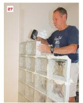
The next day, the author begins by attaching another panel anchor to the bathroom wall for reinforcement (24). He adds mortar (25) and then spacers for the next course (26). With four courses of the block wall completely solid, he continues installing the next few courses (27).
