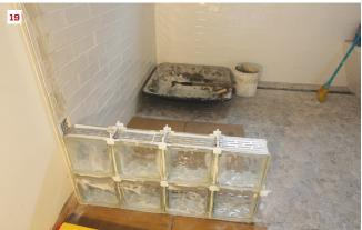
After installing two courses, the author installs a stainless steel panel anchor (which comes in 16-inch lengths) to tie the glass block to the bathroom wall framing. He bends one end of the anchor, inserts the end into the pocket cut out earlier, and screws it directly to the wall framing, with the rest of the anchor resting on the block (18). He then inserts spacers for the next course (19).
