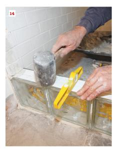
The author continues the installation of the glass block for the first course, buttering each block and tapping it into place. When the course is finished, he checks to make sure the block is in plane and on the layout lines on the floor (12). Next, he checks to make sure the course is level along its length, tapping it down if necessary (13). The third and final check for each course is leveling across the block; again, he taps the block into line if necessary (14).
