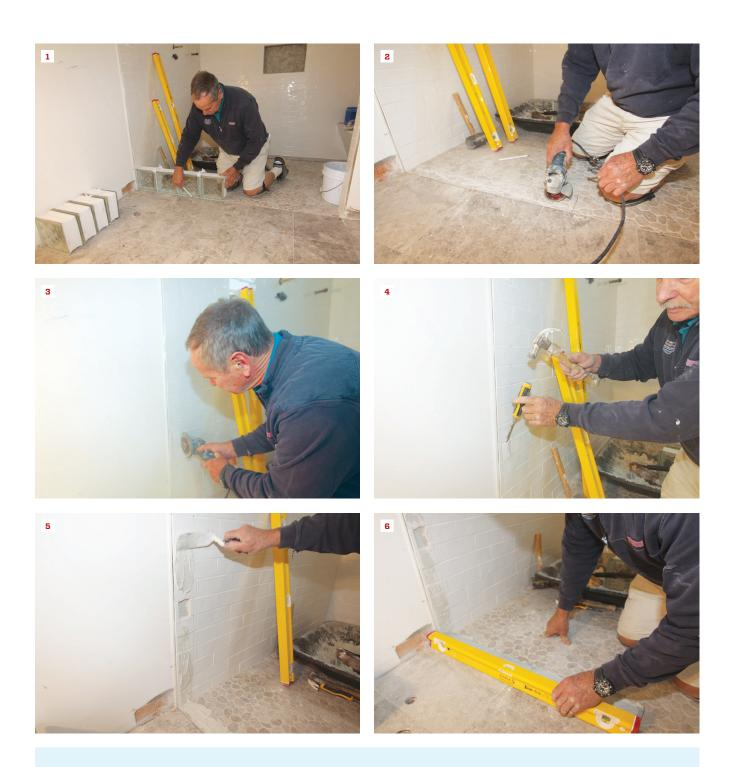
The author lays out the glass block on the floor (1) and scarifies the floor tile with an abrasive wheel on an electric grinder (2). After extending the layout up the wall and scarifying the wall tile, he cuts and removes enough tile (3) to expose the wall framing for attaching reinforcement (4). He spreads a layer of modified thinset over the tile (5) and quickly checks the floor for level (6).
