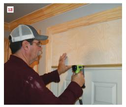
Doors that are less visible don't need the full transom treatment (10). After extending the door trim to include the transom area, the crew member removes the drywall and installs a plywood panel (11). A molding strip goes between the door and the transom area (12).
