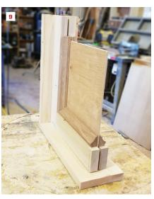
For a traditional-looking glass transom (6), the author mocked up several options. The simplest glass option captures a glass panel between two strips of panel molding (7). The second option looks more like a window sash in the transom (8). The solid panel option can be built and installed before the box goes in (9).
