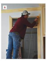
Nail together pieces of jamb material for the transom jamb (1). Install the transom jamb about ½ inch above the door jamb (2). After shimming the jamb square (3), secure the sides (4) and case the entire door and transom (5).
