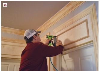
To finish off the panel, the crew member pre-assembles a decorative frame of panel molding, gluing and pinning the corners (13). Using a gauge block to space the panel molding frame away from the door trim, the crew member attaches the frame to the transom panel (14). The entire door assembly is then ready for paint.
