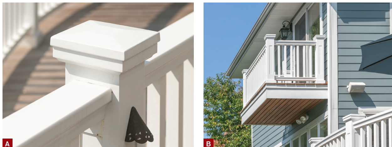
Figure 4. The author sanded the sleeves, caps, and bases and gave them a coat of 100% acrylic latex paint, then assembled all of the components on the jobsite (A). The rails were fastened to the posts with 4-inch-long screws (B).
