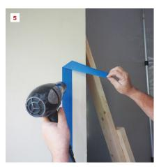
Constructed wood walls (1, 2) are the most durable way to block off an area, but aluminum or steel pole systems (3, 4) are quicker. Plastic should be taped to walls and ceilings, but stay away from finishes that could be damaged when you are removing the tape. A hair dryer (5) can soften adhesive to help prevent damage when tape is removed.
