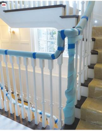
Hardwood stairs can be protected using hardboard or plywood tread covers (24), secured to skirtboards using cleats. For stair railings, the author recommends wrapping the railing in sill sealer and tape (25). Foam board works well for protecting walls (26).
