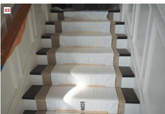
The author advises using adhesive roll plastic to protect carpets (20). Whole rooms can be protected with a sheet of 2-mil or thicker poly (21). Carpeted stairs can be covered with adhesive plastic (22, 23).
