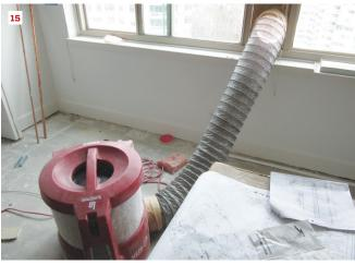
Fan choices range from a cheap box fan in the window (10, 11) to carpet dryer fans (12, 13) and dust extractor fans (14). At the top end are air filter systems (15) that come equipped with HEPA filtration. The author recommends the filter systems for situations where blowing dust out of the window would create a nuisance for neighbors.
