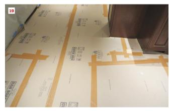
The author advises taping over HVAC supply registers (16) and taping filters over return registers (17). For protecting wood floors, he advises starting with a base layer of tacky felt (18) and adding an impact-resistant layer of durable sheet goods over the top of that (19).
