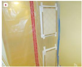
A wood screen door or demoed interior door (6) makes a good dust containment door. Other options include zipper systems (7) and commercial doors (8), which tend to be expensive. Tape furnace filters to holes in the plastic (9) to control dust while relieving air pressure from wind.
