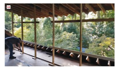
As the roof went up, the vertical supports footed against stops nailed to the dormer floor (11). The crew continued the lift in increments according to the lifting height of the jacks (12). When the supports were plumb and in contact with the outermost stop, the roof was at the proper height (13).
