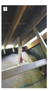
The crew cut the rafters at an angle to eliminate binding as they lifted the roof (5). Initially, they used T-shaped lifting posts between the jacks and the rafters (6). When the jacks had reached the maximum distance that the crew could lift in one shot, temporary supports held the roof while the jacks were placed on 2-by scraps for the next lifting stage (7).
