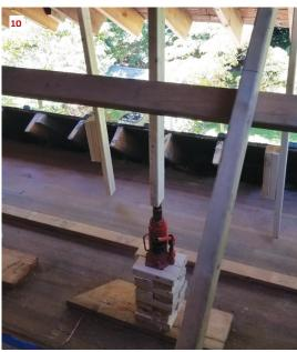
The author devised movable "jacking boxes" to hold the posts as the jacking progressed (8). After each lifting cycle, the crew installed temporary supports until the jacks could be reset (9). Instead of cutting new support posts for every lift cycle, they stacked cribbing made from 2-by scraps under the jacks (10).
