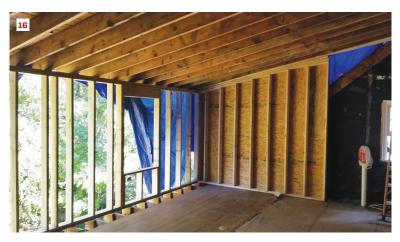
After raising the roof into position, the crew removed the bottom sections of the existing rafters (14). Using a laser level, they laid out and cut the birdsmouths for the dormer wall (15). The crew installed squash blocks along the floor joists to support the plate for the dormer wall (16). They also built and raised cheek walls at the ends of the dormer.
