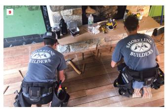
Once the crew has tacked every third row in place, one person makes a cut list for the infill boards (6). The crew cuts the infill boards and racks them between the tacked boards (7). Wedges straighten the infill boards and keep the gaps consistent while a crew member tacks those boards in place (8). Erasable white chalk lines keep the nails in a perfectly straight line (9).
