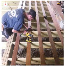
The system for installing every third board works well for long runs of decking (1). The crew snaps layout lines across the joists for every third row (2), as well as lines down the middle of each joist for nail alignment (3). Then they lay the boards down (4). After predrilling, a crew member tacks the decking on the snapped lines (5).
