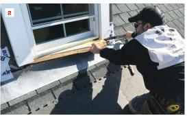
The wood sill had been in good shape when the author originally installed the replacement window and new casing (1). Since then, however, the sill had rotted and needed to be replaced (2).
