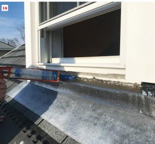
While the window opening had been properly flashed and waterproofed at the time of the replacement window installation, the author air-seals the opening by applying low-expanding foam before installing the sill (13). After the foam insulation cures, he applies a thick bead of clear silicone sealant to bed the sill in place (14).
