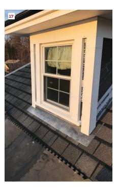
The author carefully slides the new PVC sill into position below the replacement window and the side casings (15). To lock the new sill in place, he drives galvanized screws from the edges of the casing and into the horns of the sill (16). The screw heads will be hidden by the siding. With the corner boards installed, this dormer is trimmed and ready for siding (17).
