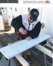
To make the sill stock, the author rips two pieces of 3/4-inch-thick PVC sheet stock (3). He applies PVC cement to both mating surfaces (4) and then drives screws to join the two sections together while the
