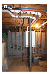
Condensate from a condensing boiler drains into a reservoir and is then pumped safely to the outdoors (1). With relatively low exhaust temps, the flue can be a plastic pipe with a high-temperature rating (gray) (2). This jurisdiction requires rated pipe for just the first 5 feet from the boiler.
