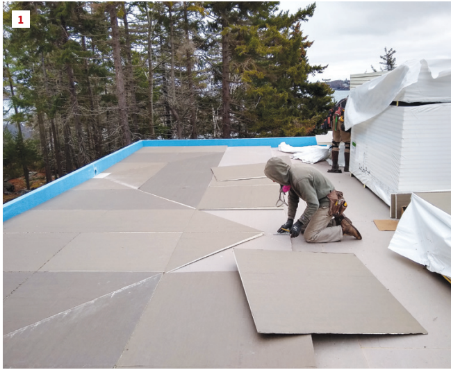
The crew builds the roof up with tapered sheets of foam, constructing valleys that lead to scupper locations in the downslope parapet wall (1). The foam buildup is fastened down with long FastenMaster screws (2).
