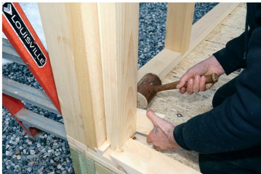
The crew fabricated the mortised and tenoned pieces in the shop, then fitted the frame together on site. The resulting joinery will be visible to summer lodgers when the rustic cabins are in use.
