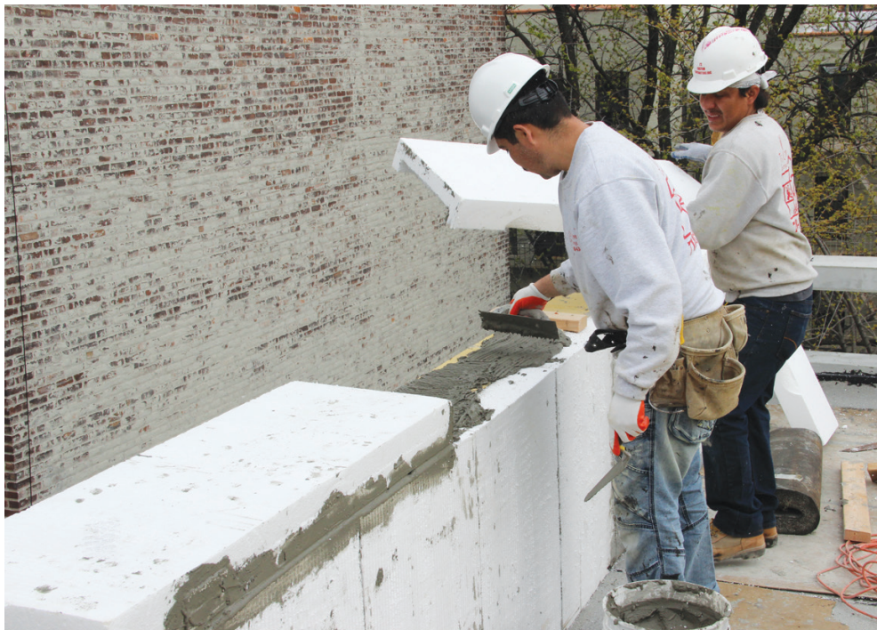
Parapet walls for low-slope roofs can be insulated with a rigid-foam wrap that integrates into the wall insulation and the roof insulation of the building, as shown here in a Passive House project from 2016.
