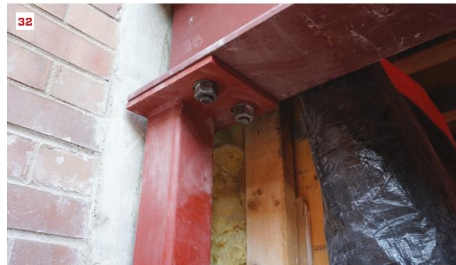
Once the structural mortar cures, the crew drills holes for  $\frac{5}{8}$ -inch attachment bolts, which are epoxied in place per the engineer's specifications (29). After the epoxy cures, the crew threads nuts onto the bolts and cuts the ends with a grinder (30). Three bolts secure the right-side base (31), and hardened steel bolts attach the tops of the columns to the support beam (32).
