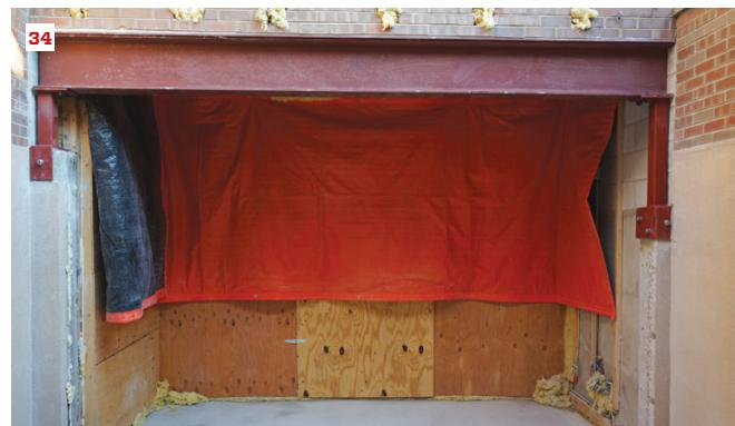
When the crew finishes installing the columns with the weight of the masonry wall loaded onto the new beam, they dismantle the shoring that supported the beam and wall. After removing the beam clamps, they back off the adjustment screws on the shoring towers (33). With the area cleaned, the space is ready to be roofed and weathered in to expand the basement living space (34).
