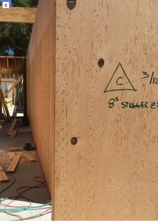
Tight edge nailing that matches the plans' shear wall schedule and a ½-inch gap are details that a building inspector will look for first (4). The nailing schedule can vary from wall to wall, so some framers mark up panels so it's clear to the crew exactly what the nailing should be. Here (5), 3/12 refers to edge and boundary nailing every 3 inches and nailing in the field every 12 inches along studs.
