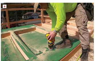
For the required connection of a shear wall to the roof structure, the author uses a Quik Stick to drive structural screws through the top plate into rafters (6). He typically installs shear panels on the deck before standing walls (7), sheathing over window and door openings and routing them out afterward (8).
