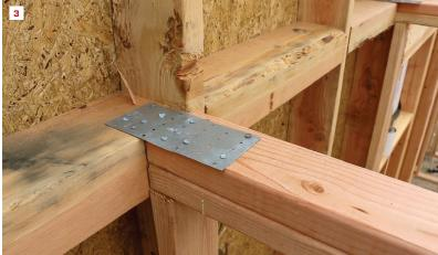
One advantage to OSB is the availability of lengths over 8 feet. Here (2), 4x10 sheets vastly simplify the shear wall on side walls. The author balloon frames gable-end walls and installs 4-by fire blocking for easy nailing of the tight edge nailing required for the shear panel (3).
