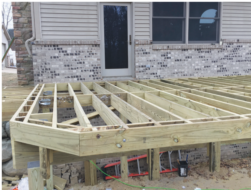
Figure 1. Vertically oriented for drainage, blocking has been added to the deck framing in preparation for installing a picture-framed border.
