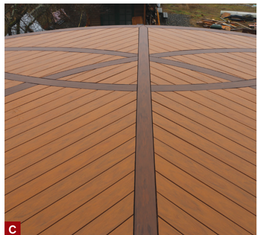
Figure 5. Special heating blankets make synthetic decking hot enough—around 220°F—to be pliable; here, Jeff Blotsky of Artistic Decks molds the hot decking around a wooden form (A). Once the boards cooled, he used them to create the unique curved picture-frame borders and inlays on this stylish deck (B, C).
