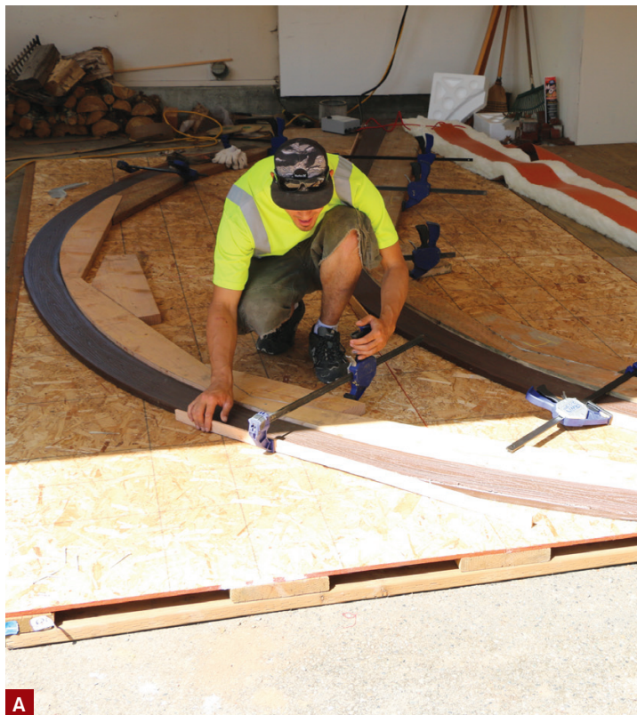
Figure 5. Special heating blankets make synthetic decking hot enough—around 220°F—to be pliable; here, Jeff Blotsky of Artistic Decks molds the hot decking around a wooden form (A). Once the boards cooled, he used them to create the unique curved picture-frame borders and inlays on this stylish deck (B, C).
