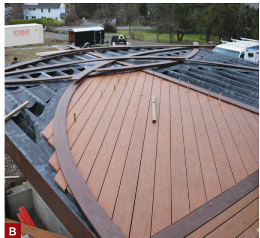
Figure 4. Ipe decking installed in a herringbone pattern adds an interesting twist to this wood deck's classic look (A). On a low deck (B), builder Brendan Casey framed the Brazilian teak decking with a Brazilian tigerwood inlay, fascia, and border. On another Brazilian teak and tigerwood deck, Casey installed a double picture-frame border and a matching crisscross inlay with a basketweave pattern in the center (C).
