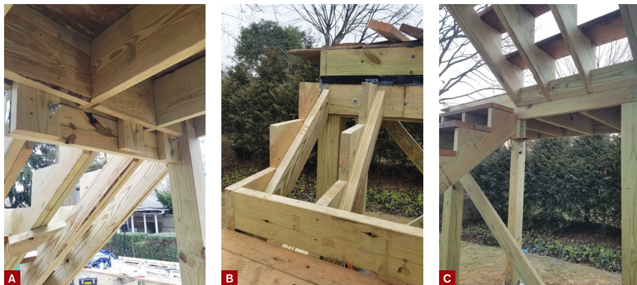
Figure 3. The stair stringers were hung from a 2x6 connected to the rim joist with vertical blocking and a combination of structural screws and Thrulok bolts (A). The author reinforced the stringers with sistered 2x6s (B) and reinforced the connection between the upper stringers and the landing platform with blocking (C).
