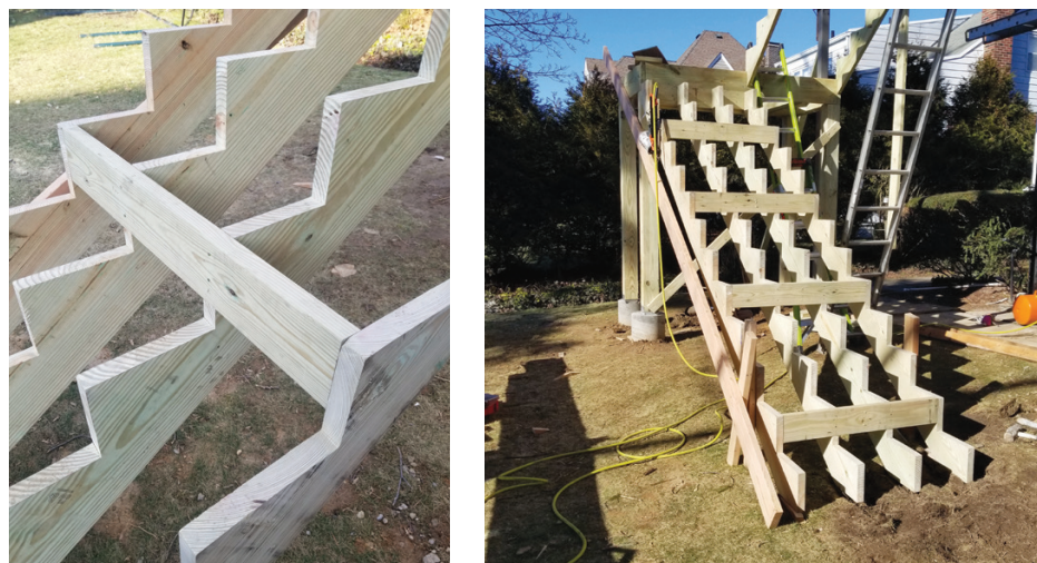
Figure 4. To make the stringers straighter and stronger, the author notched the middle stringers and installed 2x6 blocking (far left). Located every few steps, the stringer blocking keeps the tops of the treads aligned and ties the assembly together into a solid unit (left).
