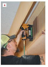
The crew began by fastening 2x4 cleats to the ceiling directly underneath an LVL beam that supports the second-story floor framing (1). After tacking MDF sides to the cleats (2), the crew added stacks of blocking (3) as they continued to build out the false beam. MDF cleats were tacked and brad-nailed to reinforce the spliced butt joints (4).
