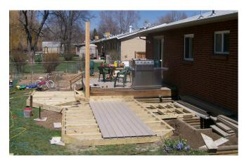
A grade-level deck doesn't need to be supported by a concrete foundation, as long as the deck is not connected to the house framing.
